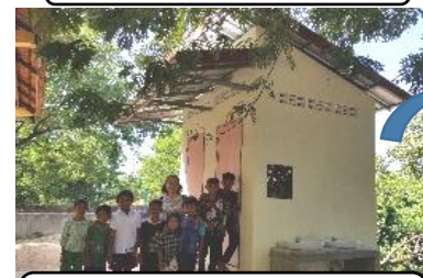
Heat-shielding container-type toilet with improved ventilation equipped with hand-washing area
